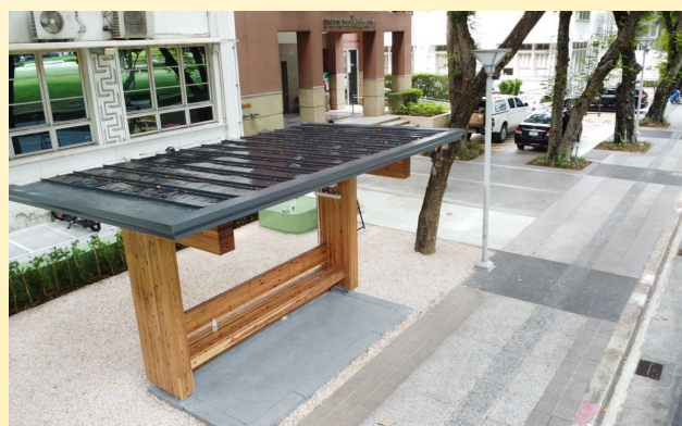
The world's first carbon-negative bus shelter in Bangkok, featuring Midsummer's thin-film solar panels.
