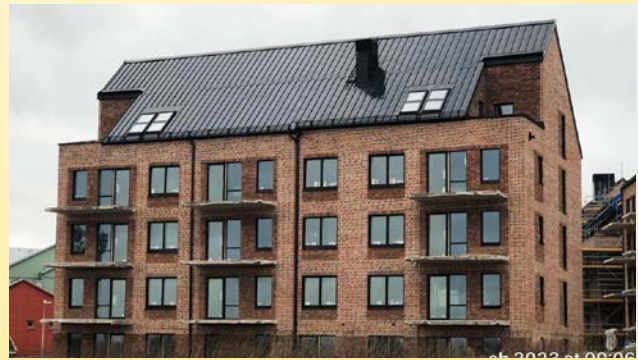
Slim installation on an apartment block in Lund, Sweden.
