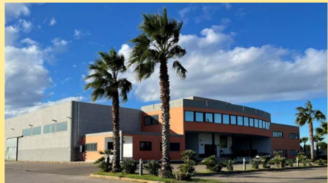
Midsummer's new factory in Bari.
